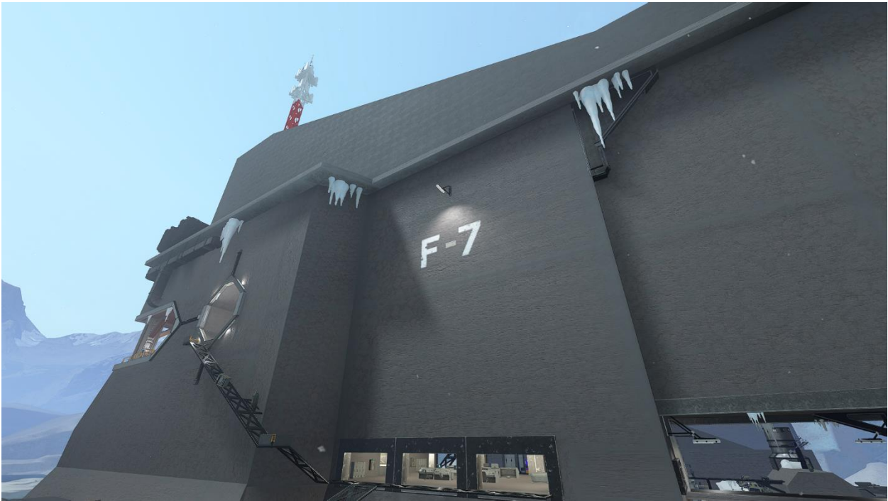
Figure 117 - Large icicles are hanging off the roof of the control building
