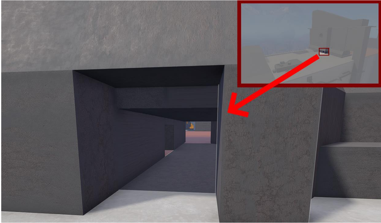
Figure 18 - Entrance into control building. Looking inward, there is an entrance to the stair well on the left wall.
