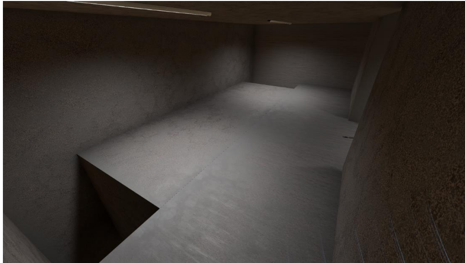
Figure 87 - The original room only had two holes to travel up and down through
